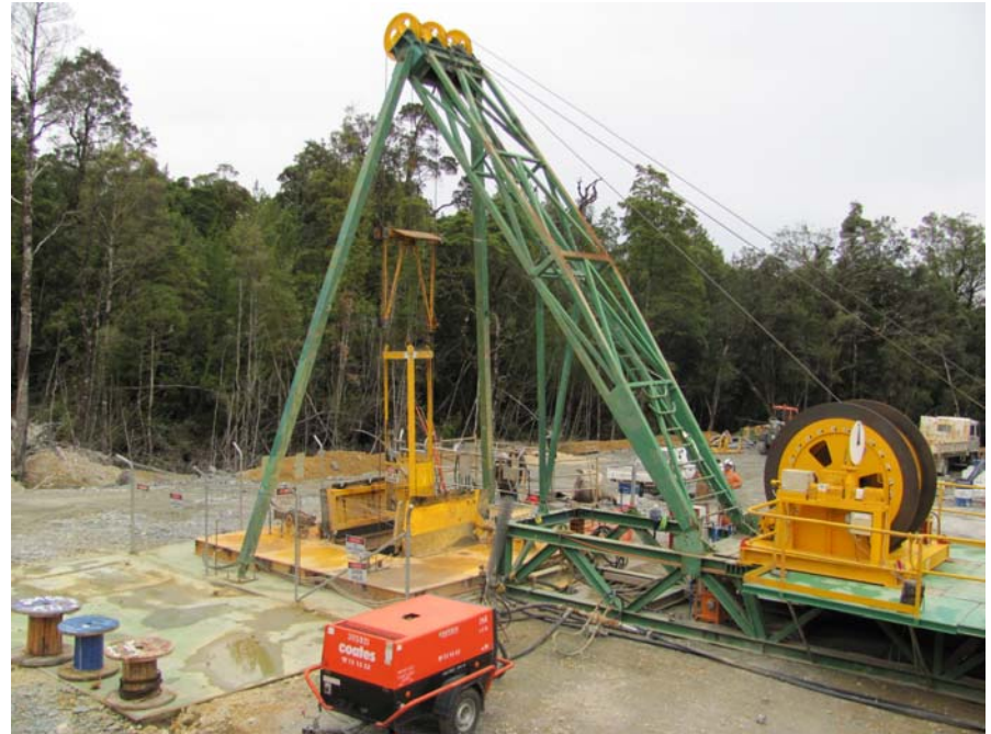
Raise bore drilling for additional ventilation shaft underway.
