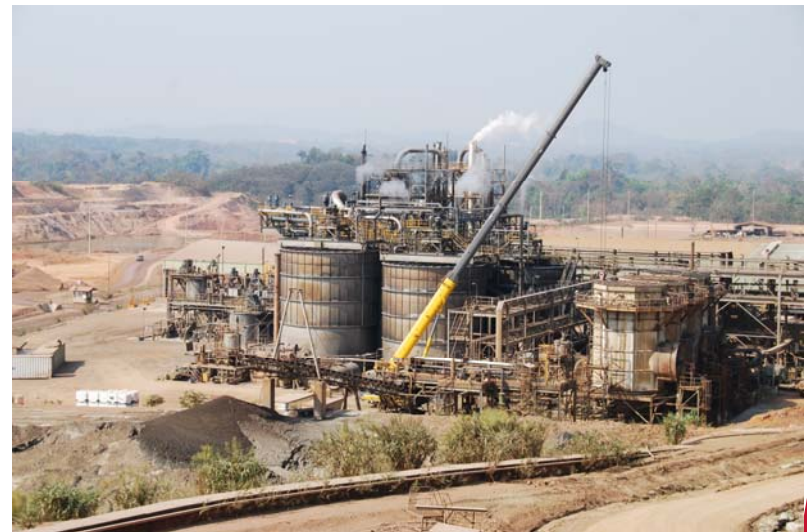
Copper expansion underway
